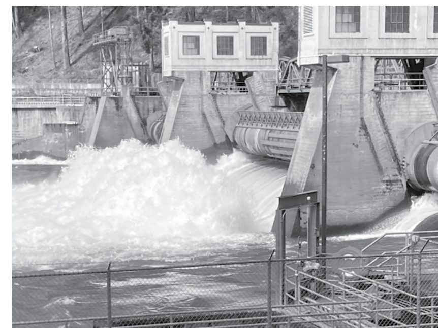
Fish killing turbulence with one gate open
